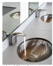
In addition, the restroom sinks were furnished with the <u>02515 electronic</u> mixers. One of the highlights of this product is the legionella – free system, which automatically dispenses a stream of water 24 hours after the last use to prevent water stagnation and the growth of bacteria.
